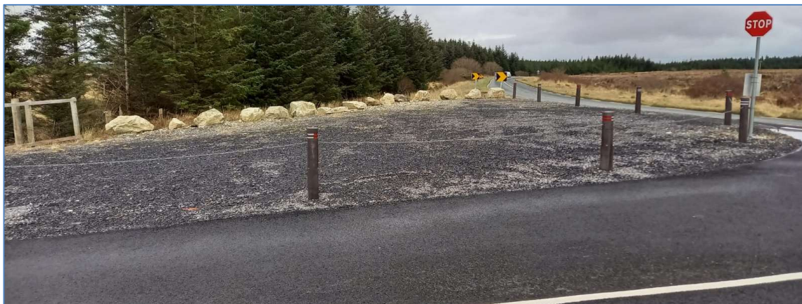
Plate 17-2 Site Access on N59 – View to East on the N59
